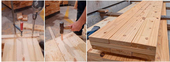
Fig. 1. Fabrication of structural-size DCLT panels.
